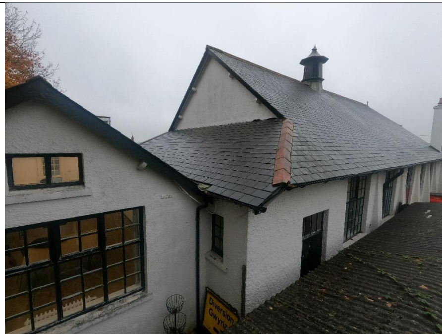
Figure 2 - A view east at the north roof
