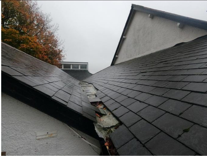
Figure 3 - Valley between north roof and rear building
