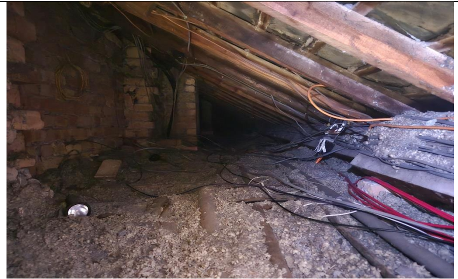
Figure 20 - Above toilets looking north
