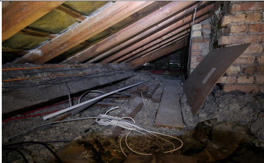
Figure 19 - Above toilets looking south
