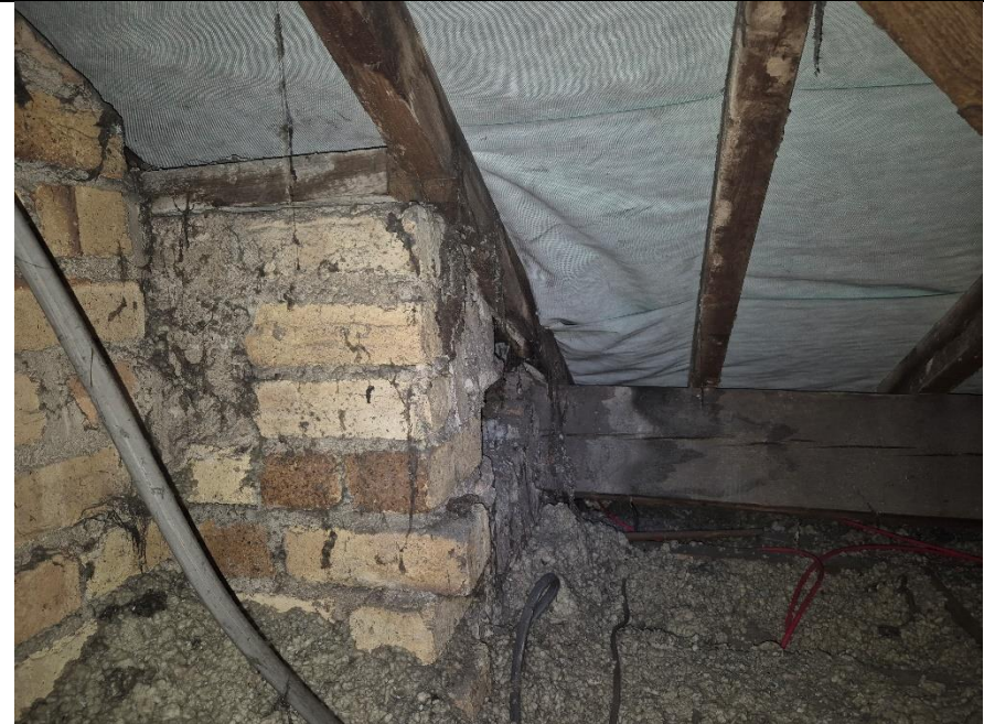
Figure 24 - Tyvek breathable membrane to reroofed area
