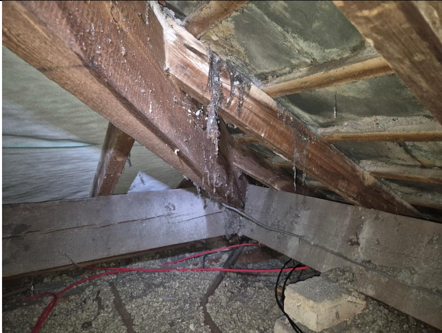
Figure 23 - North end (re-roof)
