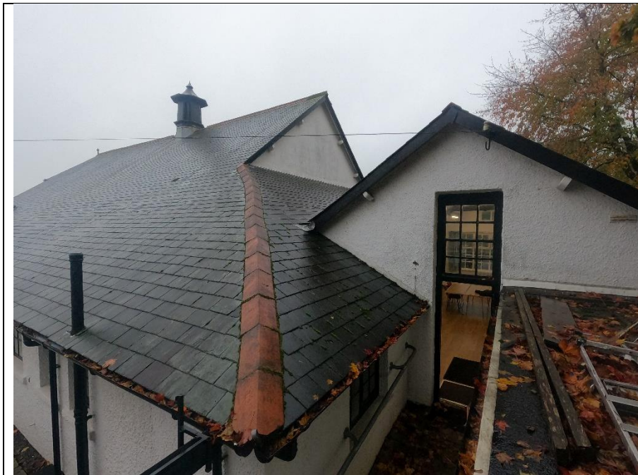
Figure 1 - A view west at the north roof
