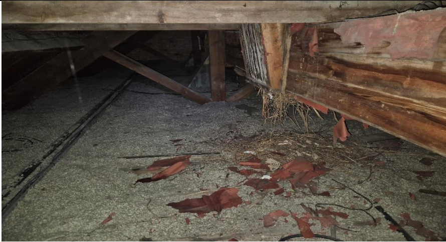
Figure 29 - Crows nests in air box vent
