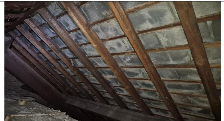
Figure 32 - Slate delamination
