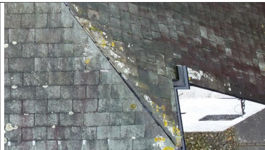
Figure 12 - Open hip joints
