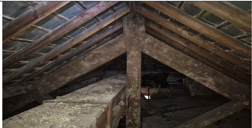
Figure 28 - Air Box looking south
